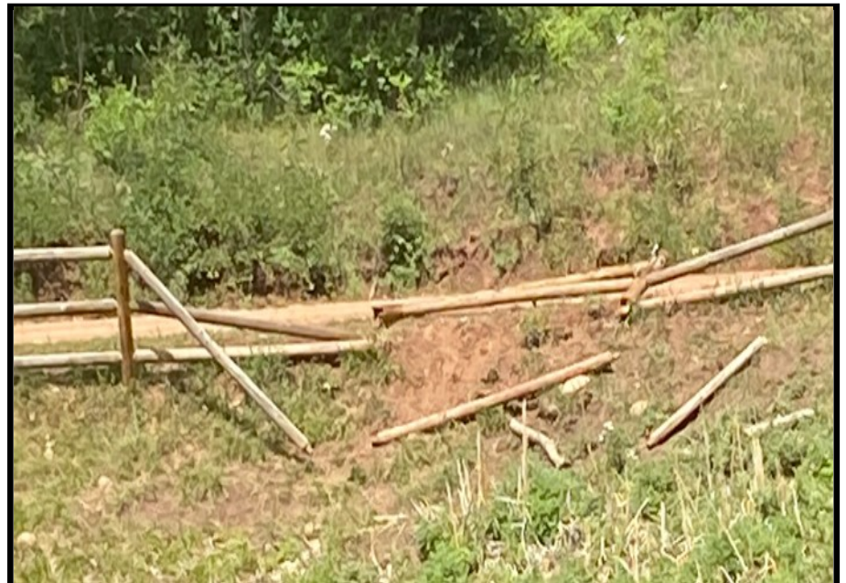
Fence damage around the lake caused by the cows grazing in the area.
